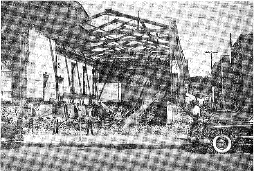
DEMOLITION OF SECOND STREET BUILDING
